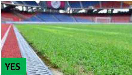
Proper drainage cover
