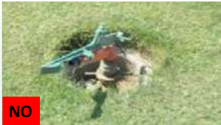
Exposed irrigation head
